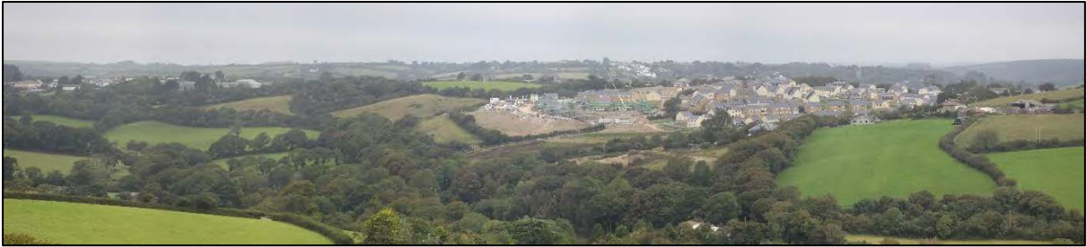
Looking north west with TL6A to the right of the image and TL18 in the background
